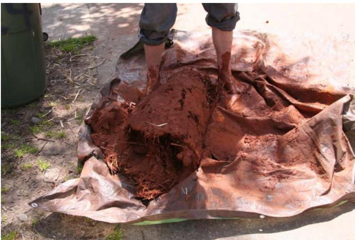
**FIGURE 1.** Mixing cob using the tarp method.
