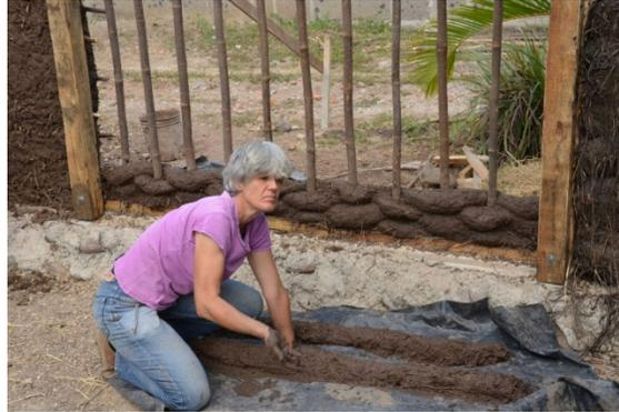
Fig 11. "snake-like" copping method around wattle frame
