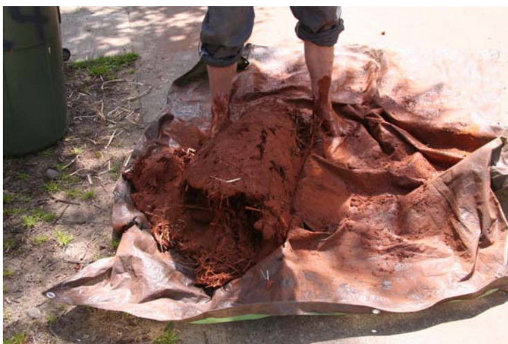
FIGURE 1. Mixing cob using the tarp method.
