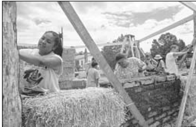
Volunteers working under the guidance of BWB to build a straw-bale hogan at Sacred Mountain Camp, New Mexico
