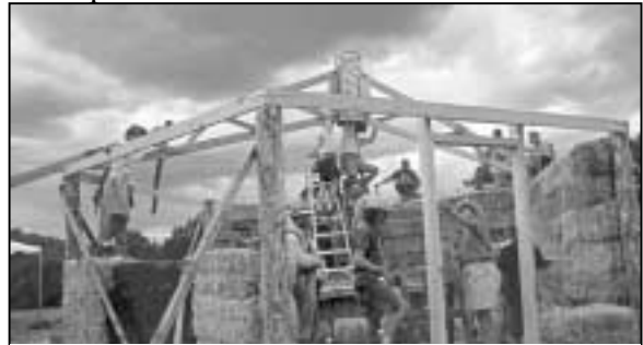
The NIYLP hogan framework in place, with straw bales going in.
