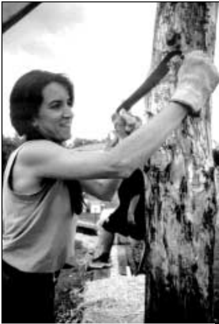
BWB organizer Susan Klinker, peeling logs for the hogan post-and-beam framework
