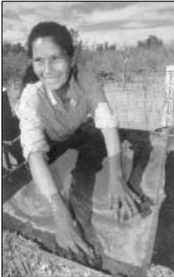
Myra Valez mixing straw-clay plaster by hand at the “Casas Que Cantan” project co-developed with local communities by BWB partner the Canelo Project
